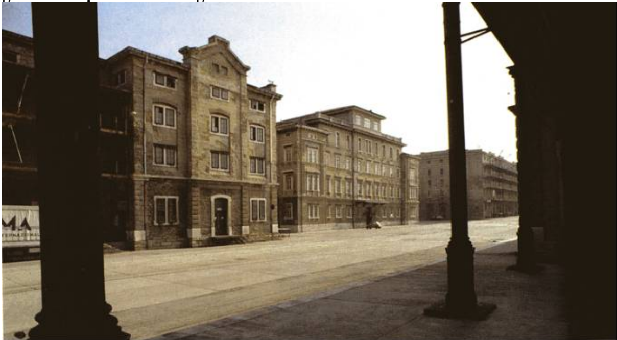
Figure 1 - Snapshot of buildings of Trieste Old Harbour
